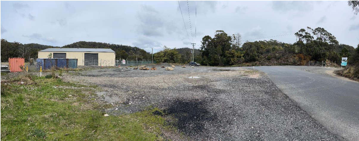
Figure 3 Existing shed and access
