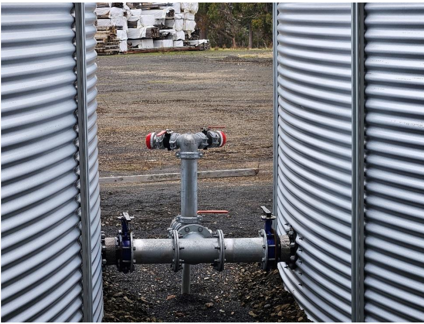
Image 5.2 – Existing standpipe and outlets
