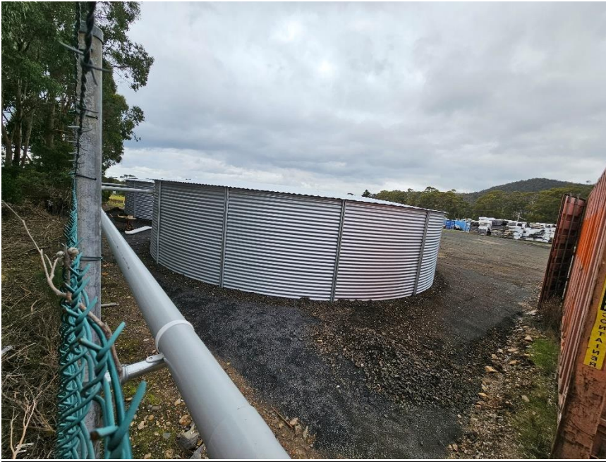
Image 5.1 – Existing static water supply tanks
