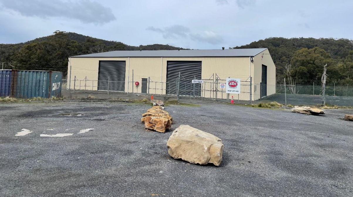
Figure 2 - Location for development – existing shed
