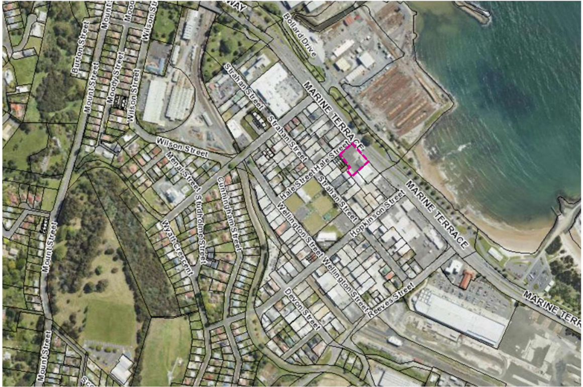
Figure 1: Aerial view of the 53-54 Marine Terrace site (Source: The LIST - www.theLIST.tas.gov.au , State of Tasmania)
