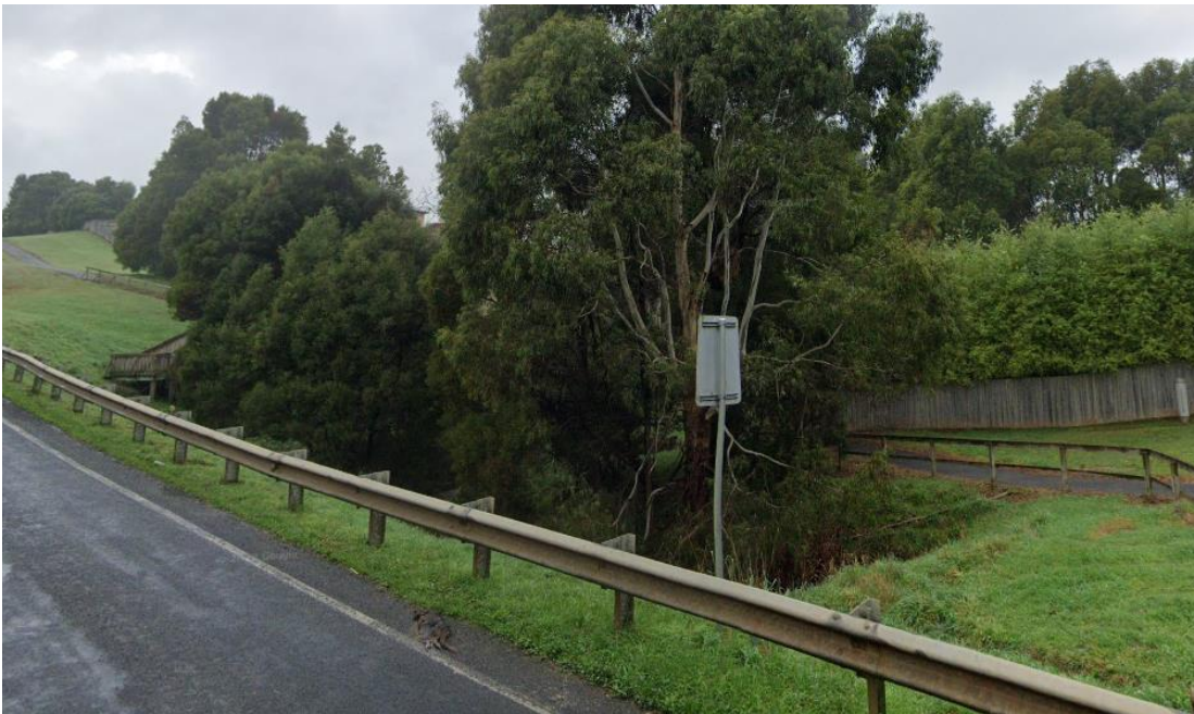
Figure 3: view of the subject development area, as viewed from Mount Street (source: google maps)
